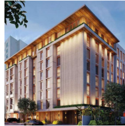
PARKSIDE Mixed-Use 206 Units, 2 Commercial Spaces 2023 - 2027
