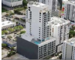
SMART BRICKELL TOWER 1 Period: 2017 - 2023
